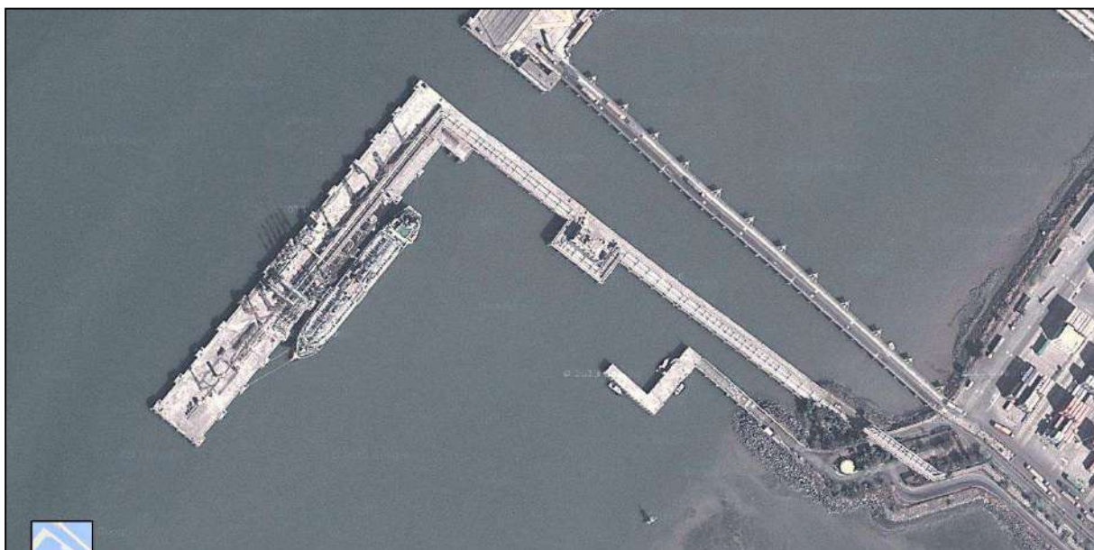
Fig 6.1 Liquid Cargo Jetty of JNPT
